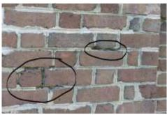
The Board of the Westover Civic Association authorized funds to repair the brick entrance way into Westover. Over the years the entrance way mortar deteriorates and is in need of repointing. This is a big expense but one that is necessary to avoid further damage. We hope
